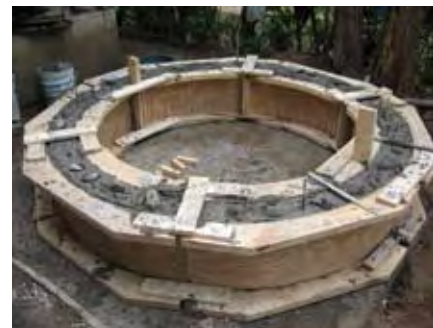
The wooden structure holds rebar, river rocks and mortar in place for it to dry on top of the concrete foundation. Once dried, the wooden forms were raised and the process continued three more times until the structure grew to about seven feet tall.
